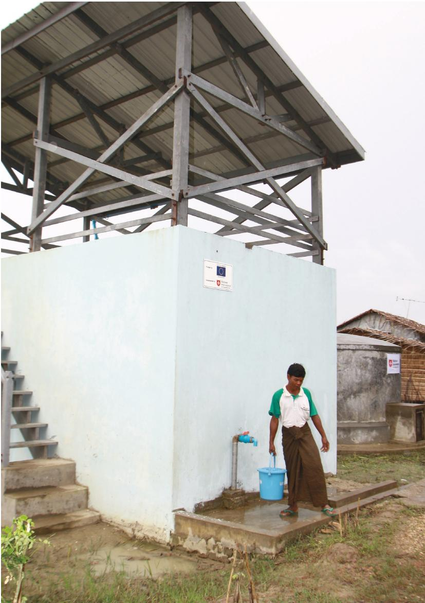
▲ Rainwater collection tank with triple function in the Ayeyarwaddy delta, Myanmar
